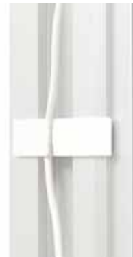
CLEAN CABLE MANAGEMENT
